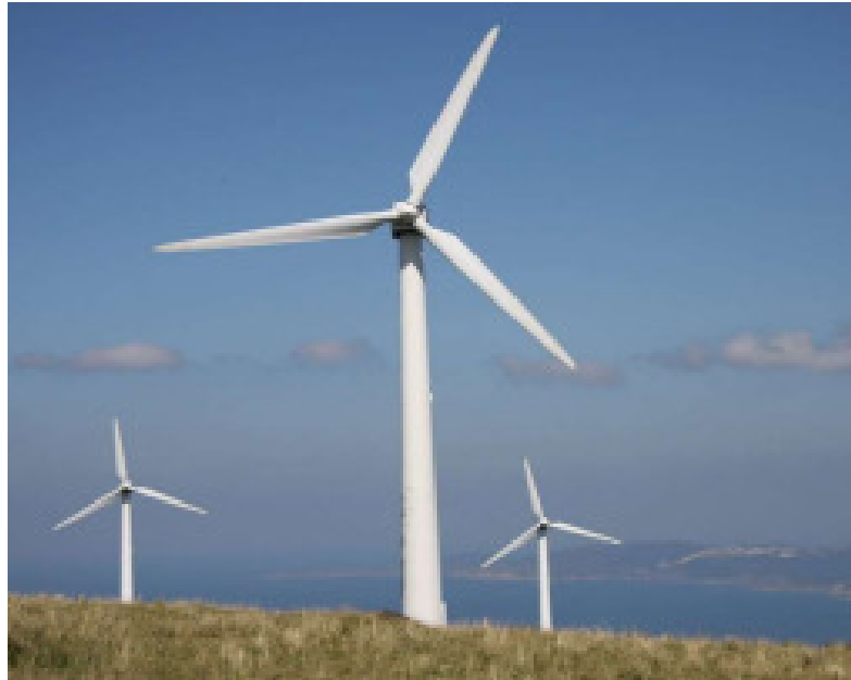
Figure 3: NEG Micon 1.50MW Wind Tower, Tubular Steel Tower, around 136m Rotor Radius. Fiberglass is used to make the blades. The whole turret is rotates to aspect the wind, and the blade of rotor can be twisted to maximize output [15].
