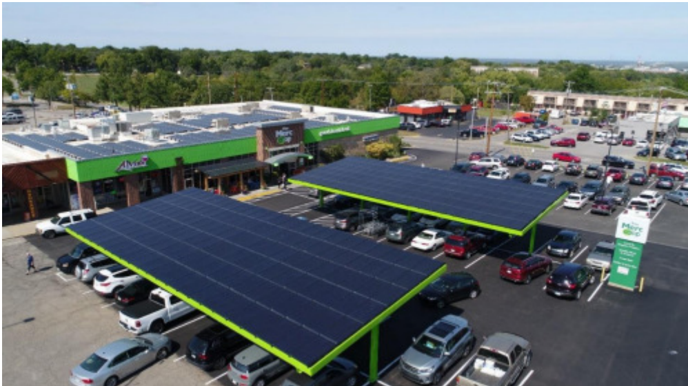
Figure 3: Demonstrate the Solar Energy Based Charging Station for Electric Vehicles in Parking Lots [12].
