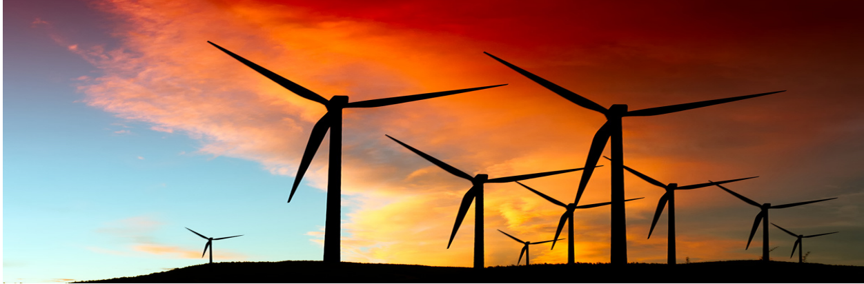
Figure 2.9: Wind power plant
