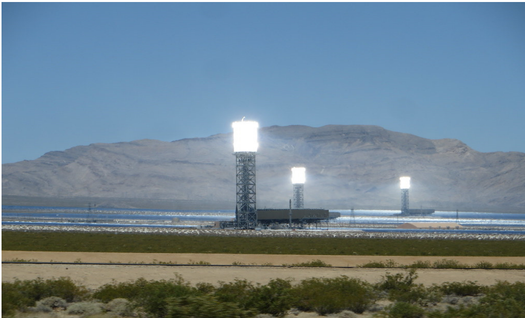
Figure 2.7: Solar power plant
