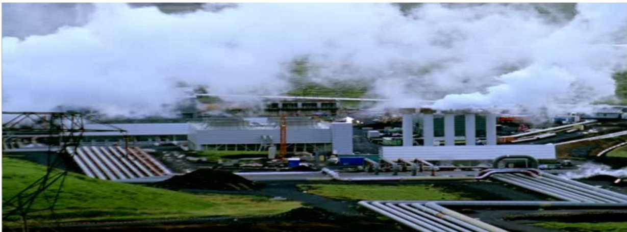
Figure 2.8: Geothermal power plant
