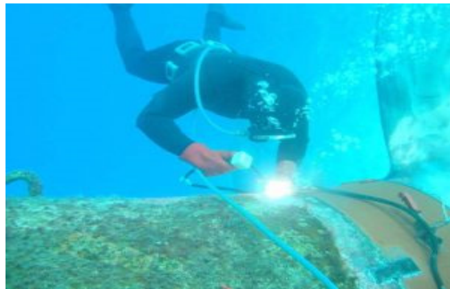
Figure 1: Representing the Under Water Welding process [Make Money Welding].
